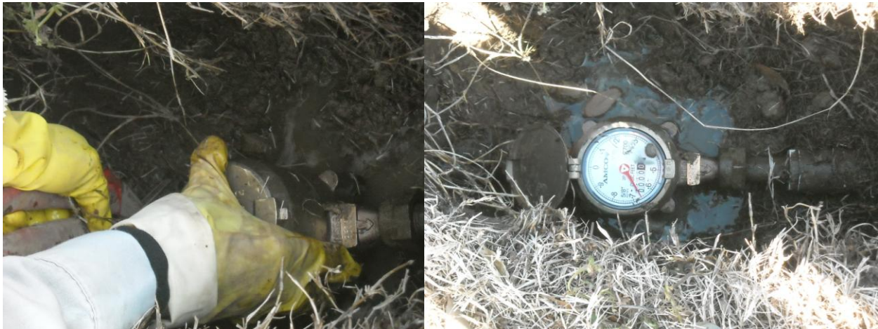
Replacement of a water meter by field forces
