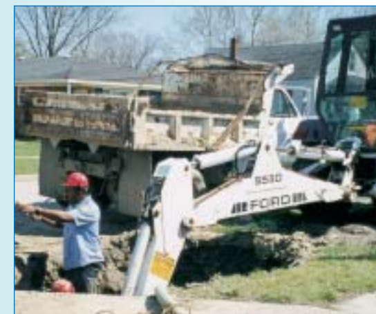
Water distribution crew making a water line repair
