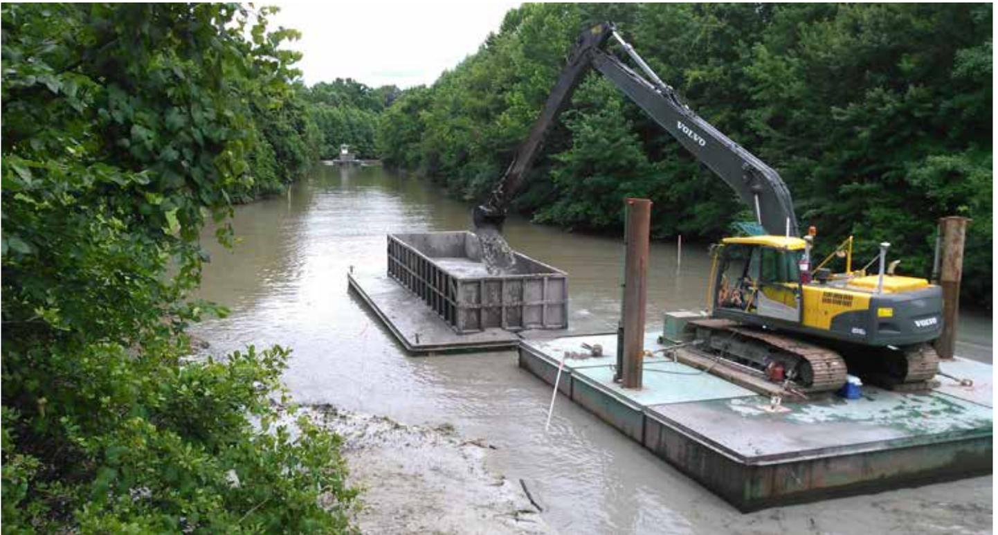
**T**he Cooper's Ditch Dredging Project is completed. The project removed more than 38,000 cubic yards of sediment and restored the ditch's bottom profile. The project came in under its \$2 million budget. Cooper's Ditch is a key element in Chesapeake's Stormwater Management Program.
